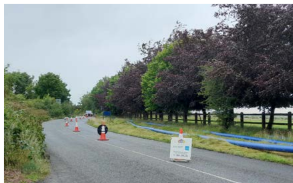
Watermain replacement works at Bracklon, Edgeworthstown
